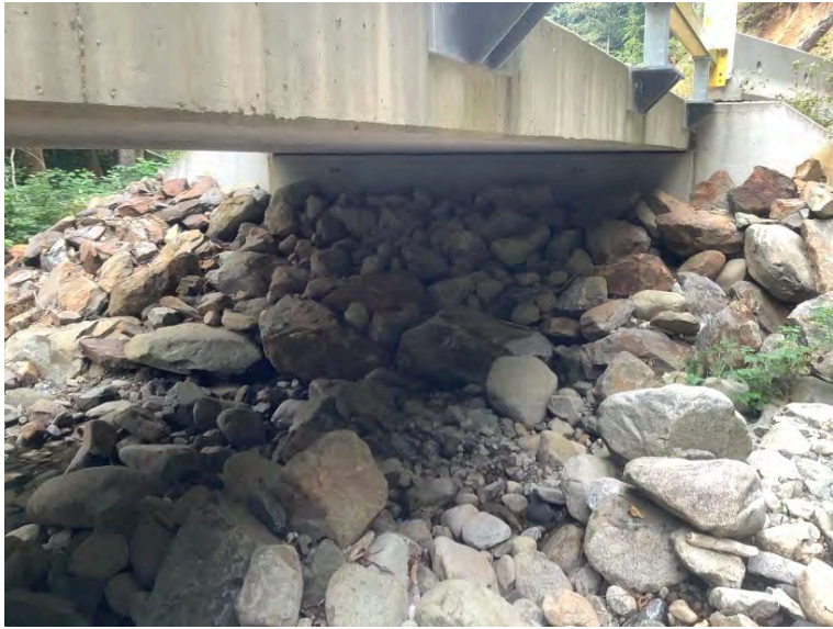
Right Bank Abutment when facing downstream
