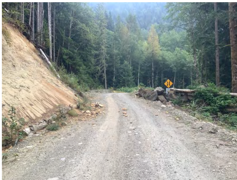
Approach from Right Bank when facing downstream
