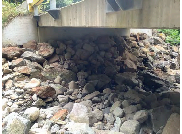
Left Bank Abutment when facing downstream
